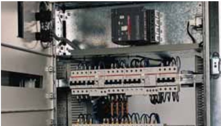
The panels for Tmax, and Emax circuit-breakers have 100mm modularity
